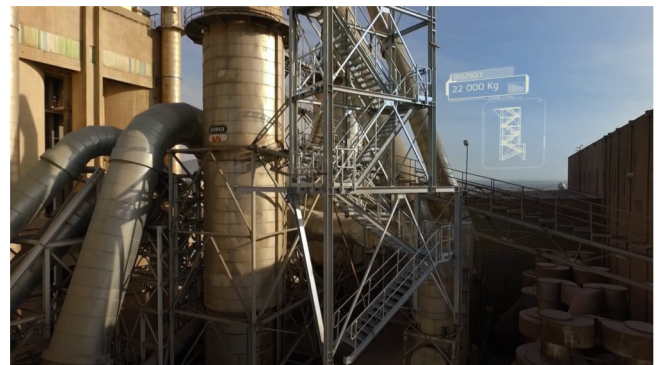
Craning and installation of a pre-fitted staircase - 22 tons
